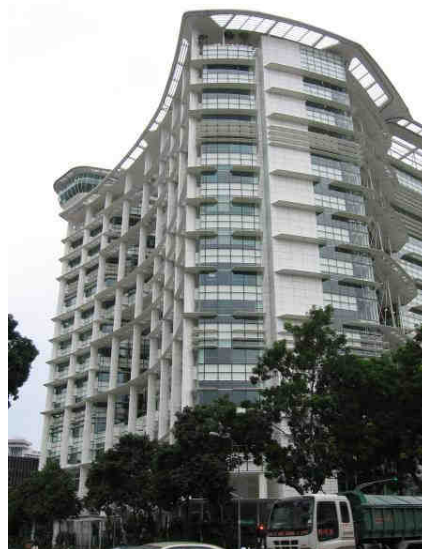
The National Library Building, Singapore – BCA Green Mark Certified
